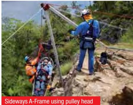
Sideways A-Frame using pulley head
